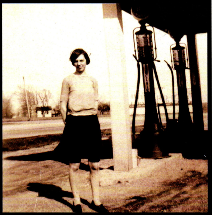
Gravity feed visible gas pumps (c. 1920) are ready to go at the filling station which is now the Club 21 on Lapeer Road.
